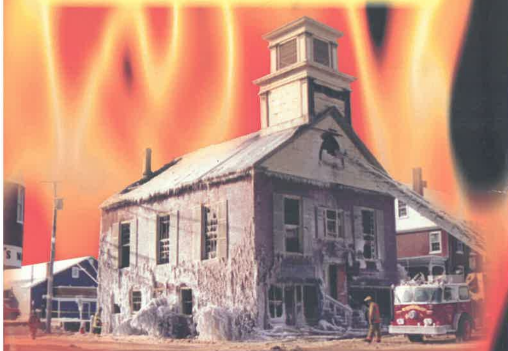
The old Baptist Church, home to the Marionette Theater at the time, the morning after the great fire, January 1, 1999. Crews remained on duty through the night, with the ladder pipe fixed in position to continue water flow. With the frigid temperatures, the entire structure and surrounding landscape was encased in ice.
