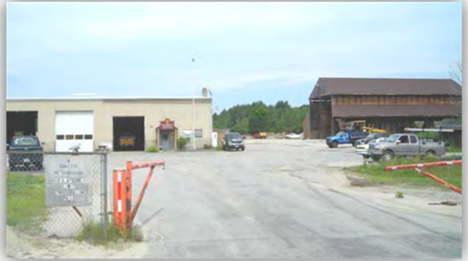
Figure 4: Highway Garage and Salt Shed
