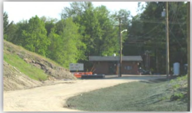
Figure 5: Water Department Building
