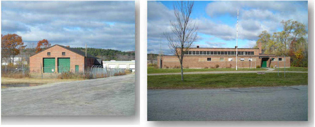
Figure 11: The Maintenance Building (left) and the Armory Building (right)
